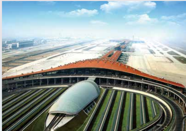
▶ Beijing Capital International Airport Location: Beijing, China Product: PCA heat pump, evaporative chillers
