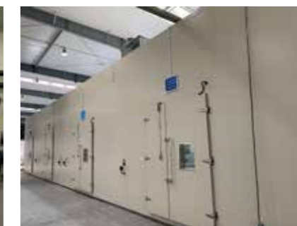
R290 A/W heat pump performance lab
