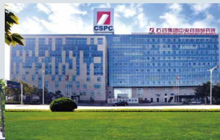
▲ CSPP Central Institute of Pharmaceutical Research Location: Hebei, China Product: Combined AC unit, thermostatic & humidistatic AC, HRV
