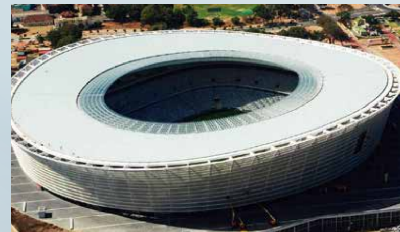
▶ Soccer City, 2010 FIFA World Cup Location: Johannesburg, South Africa Product: water source heat pump, AHU
