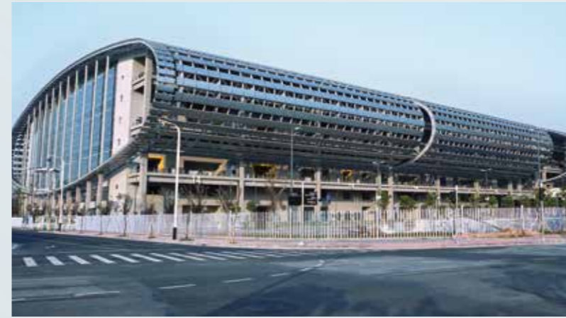
◀ Canton Fair Exhibition Center Location: Guangzhou, China Product: chillers, AHU
